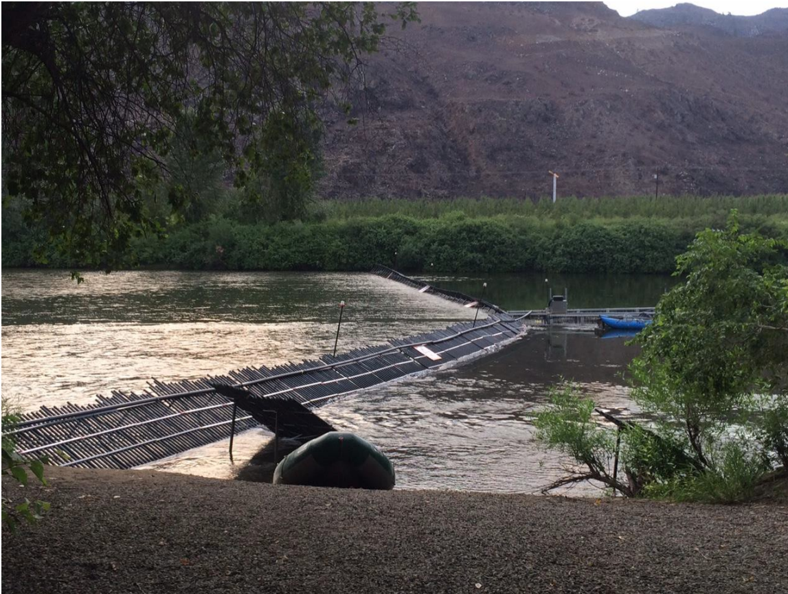
Figure 2. The deployed weir in 2014. The water deflecting panels are visible in the foreground.
