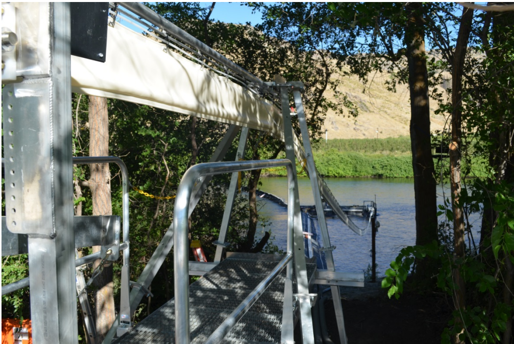
Figure 1. The configuration of the Whooshh™ tube system and the Okanogan weir trap. The tube is connected to the east, upstream side of the trap box and a stationary trailer on the east shore. Adult fish that are transported through the tube are directed into a 2,500-gallon tanker truck.
