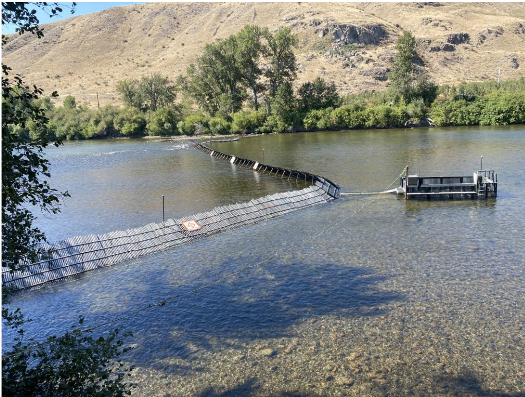
Figure 1. Lower Okanogan adult fish pilot weir, 2022. Photo taken in early September shortly after deployment.
