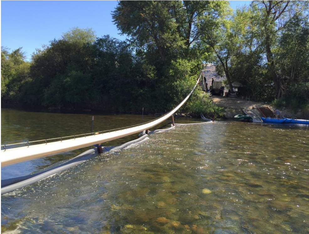
Figure 8. Whooshh™ fish transport system installed at the Okanogan weir. Photo taken from the gangway at the trap.
