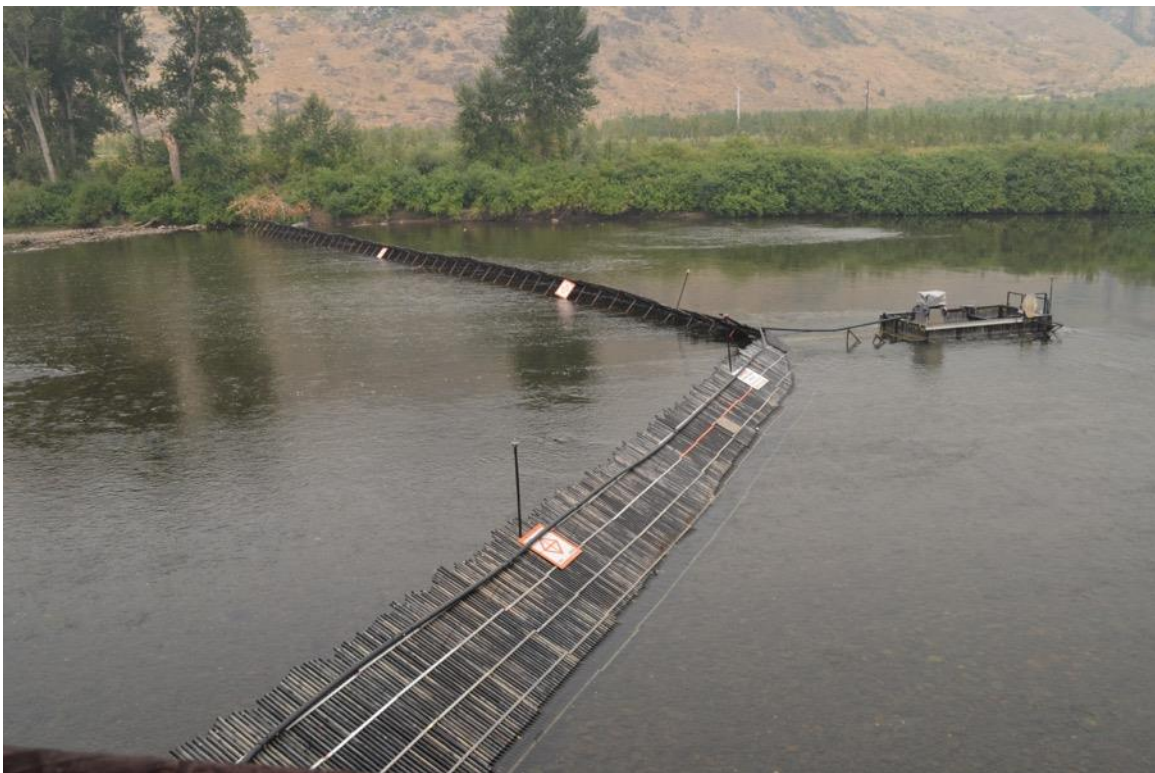
Figure 6. Lower Okanogan adult fish pilot weir, 2018. Photo taken in mid- August after deployment.
